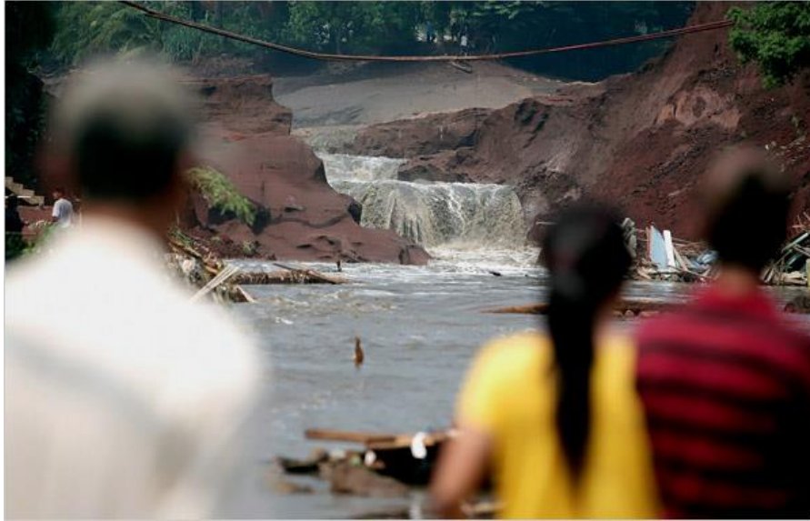
Figure 8 The Situ Gintung dam falls apart in Jakarta, Indonesia.
